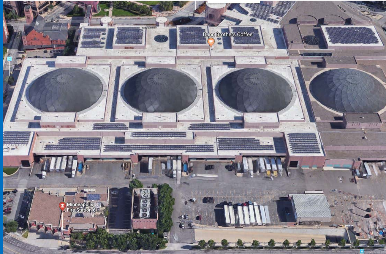
Minneapolis Convention Center – 600kW Minneapolis Fire Station 6
